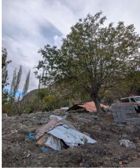
The aftermath of recent floods
