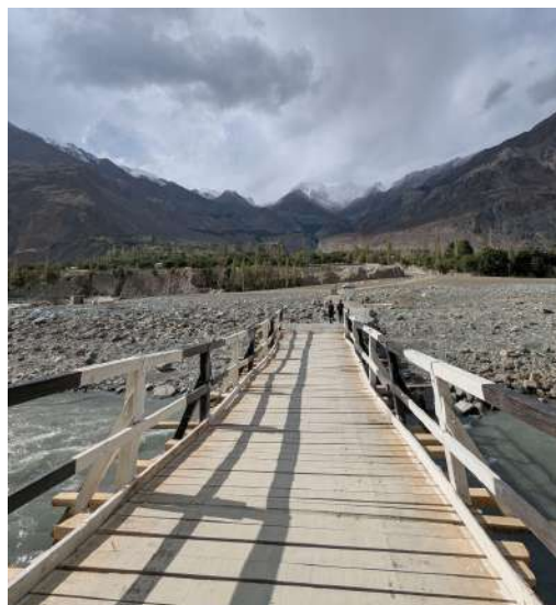
The temporary bridge constructed by local volunteers
